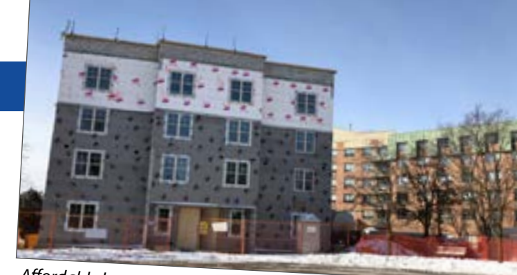
Affordable housing development underway at Water Street
